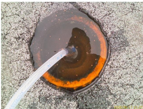
Run-off with a water column
